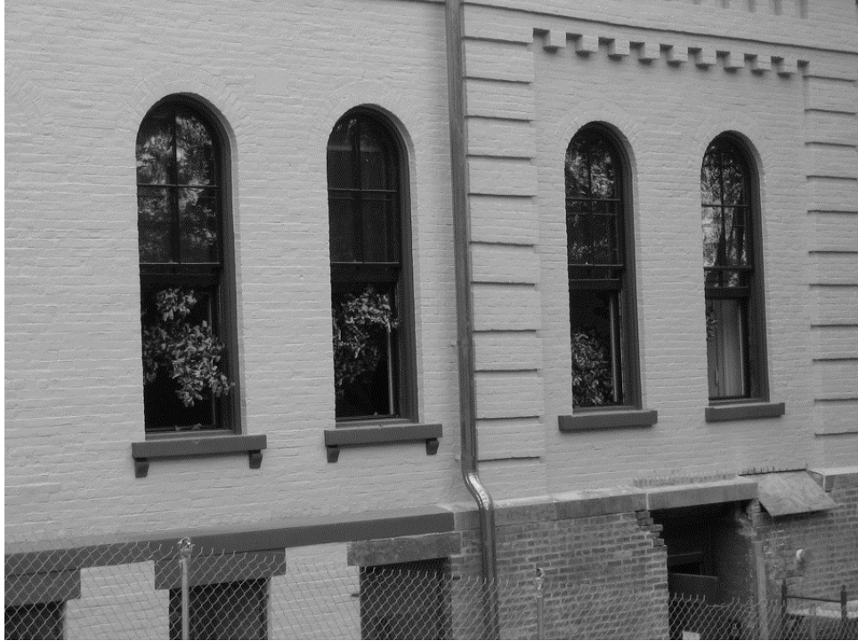
Figure 11. West Hall gallery view (exterior).
