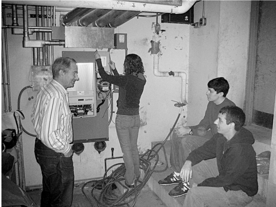
Figure 3. Installation of the Heliotronics sensor system.
